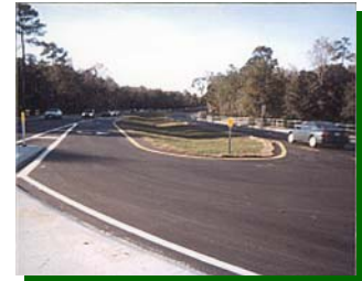
View of completed roadway
