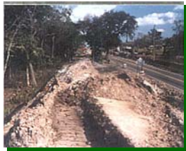
View of surcharge area I looking East
