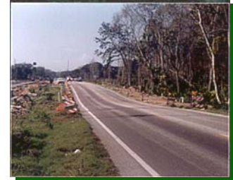
View looking west at settled portion of existing roadway
