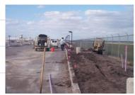
An overflow parking area, for 1,100 additional vehicles, was also built as part of this project. The overflow lot consisted of paved driving lanes with parking surfaces constructed of sod on top of geotextile-stabilized subgrade soil.
